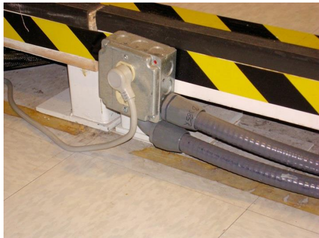
Figure 2-4: Computer Flooring Obstruction
