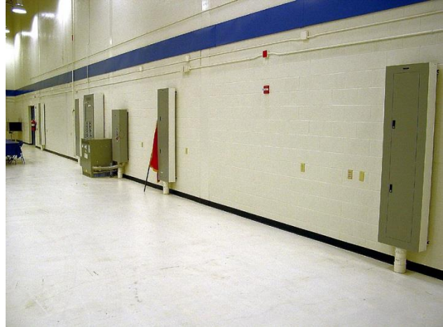
Figure 2-3: Electrical Transformer Obstruction
